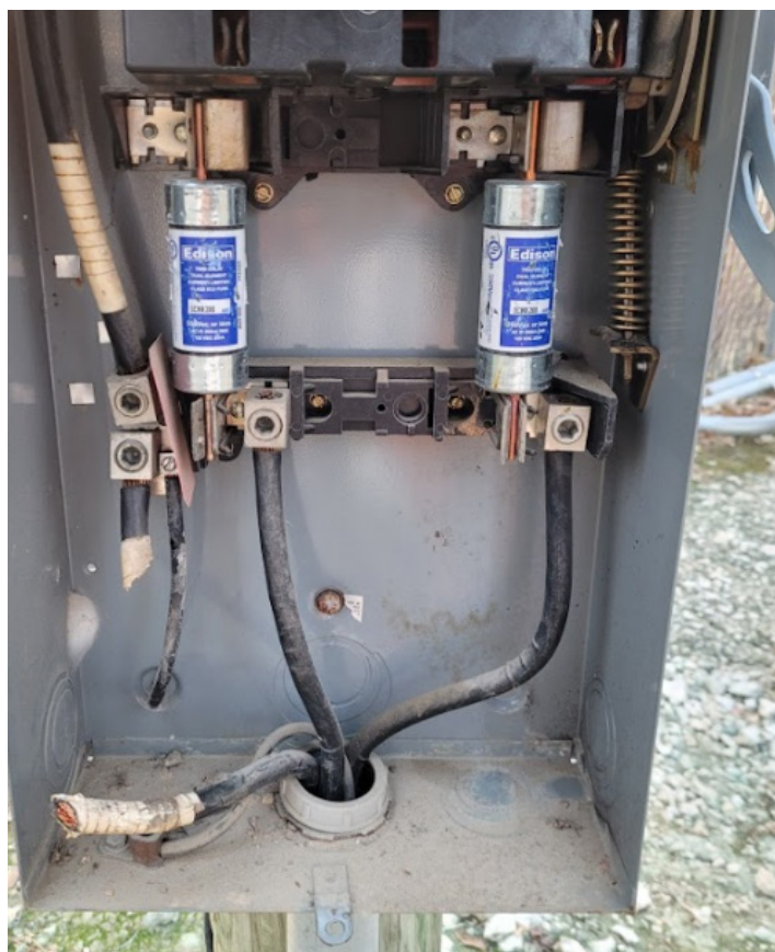
Left: Successful cuts and theft of wire in equipment cabinet. Top right: Cuts to wires on utility pole in conduit. Bottom right: Cuts to wires on utility pole in cabinet.
