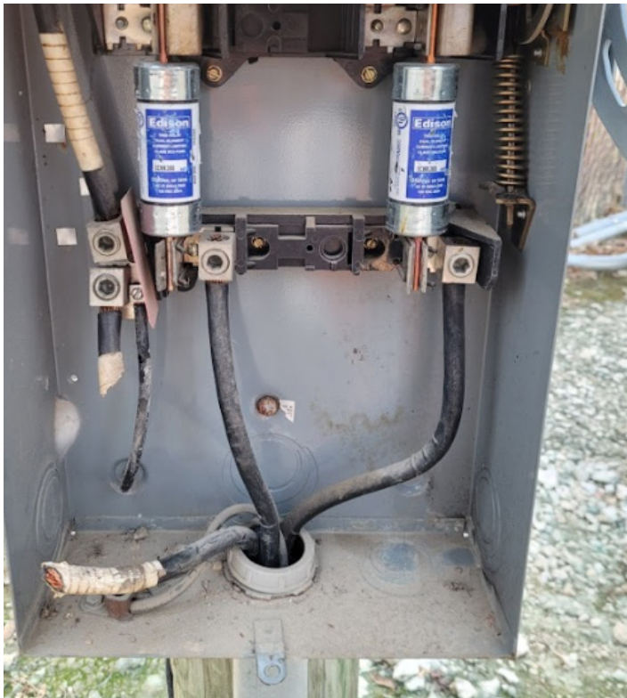
Left: Successful cuts and theft of wire in equipment cabinet. Top right: Cuts to wires on utility pole in conduit. Bottom right: Cuts to wires on utility pole in cabinet.
