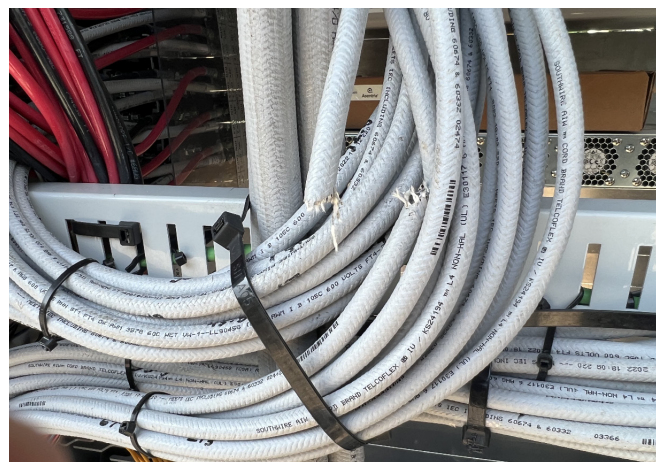
Left: Successful cuts and theft of wire in equipment cabinet. Top right: Cuts to wires on utility pole in conduit. Bottom right: Cuts to wires on utility pole in cabinet.
